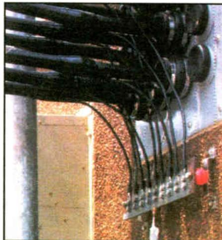
Figures 3 & 4: Left: RTV compound plugs the entrance of this PVC pipe used to protect ground wires. Right: The PVC pipe also works well at the base of a tower, protecting ground wires.
