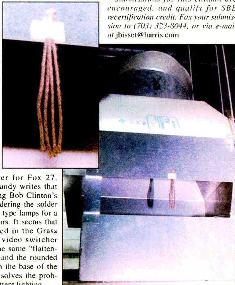
Figure 3: Here's a simple, effective way to ensure that positive outside air pressure is not defeating your cooling system.
