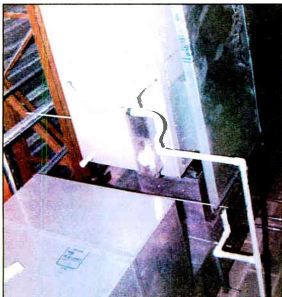
Figure 2: The extra expense of a condensate drip pan can save thousands of dollars should the drain clog.
