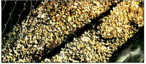
Figure 6: Ground radials are shown attached to the copper ground screen at the base of the tower.
