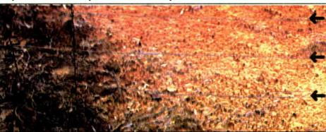
Figure 7: These ground radials, indicated by arrows, are exposed.
