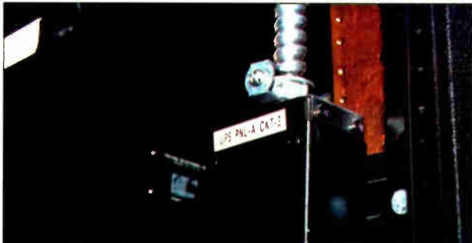
Figure 1: Mark power strips with panel and circuit designators.
