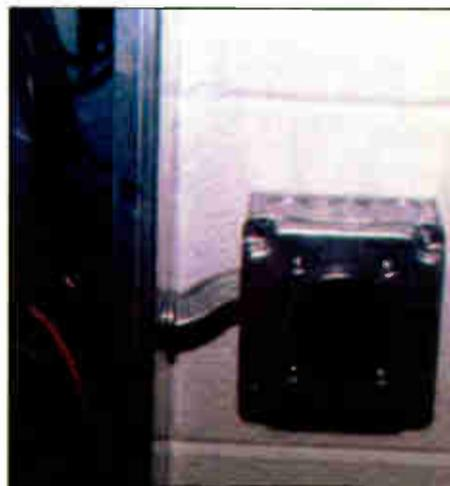
Figure 2: A spare 220VAC outlet box will speed installation of an emergency low-power transmitter.
