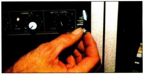
Fig. 2: A modified bolt can support equipment in a rack
