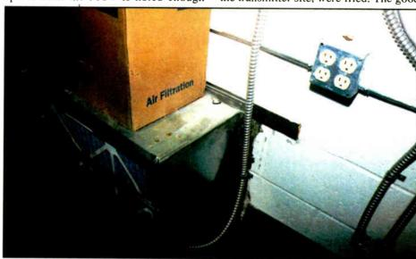
Fig. 3: Use duct tape to seal filter entries
