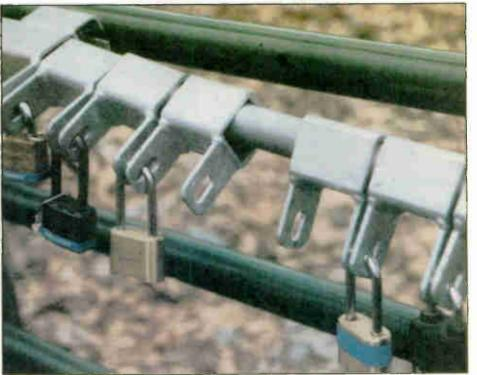
Fig. 2 shows how the access bar slides out once a lock is removed.
