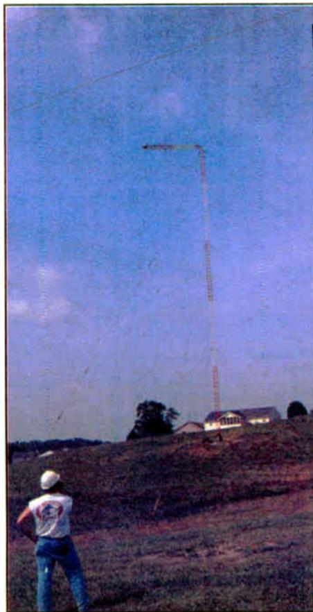
Fig. 2: Professionally dismantled, the tower is allowed to fall on itself.
