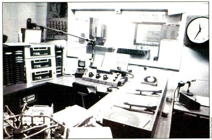
WPEN Studio B was used for most programming during the day. This photo is from 1972 after the air talent obtained the right to play their own records. The engineer controlled levels and played commercials or other audio sources. Cart machines were for jingles. The miniconsole for the turntables is a passive mixer built by the engineering staff. The window looks into MCR.
