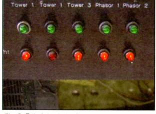
Fig. 2: Tally lights help diagnose contactor failure.
