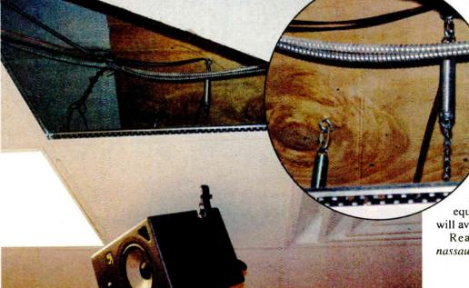
Fig. 1: You can isolate a studio speaker using springs.
