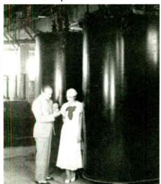
The 11-foot modulation transformers used in the WLW 500,000 W plate-modulated transmitter. Image courtesy Charles Stinger, AWA.
