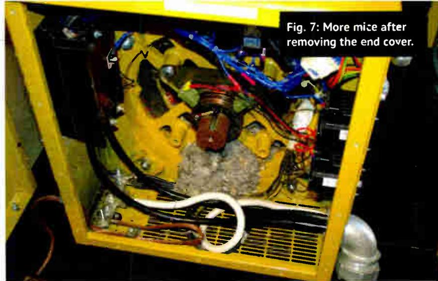
**Fig. 7: More mice after removing the end cover.**
