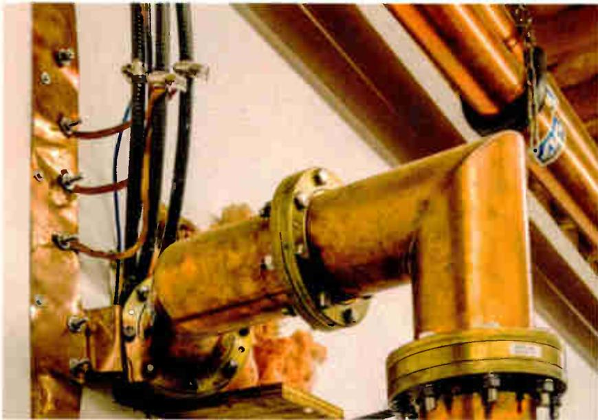
Fig. 5: Cables tied to ground at a building entrance.
