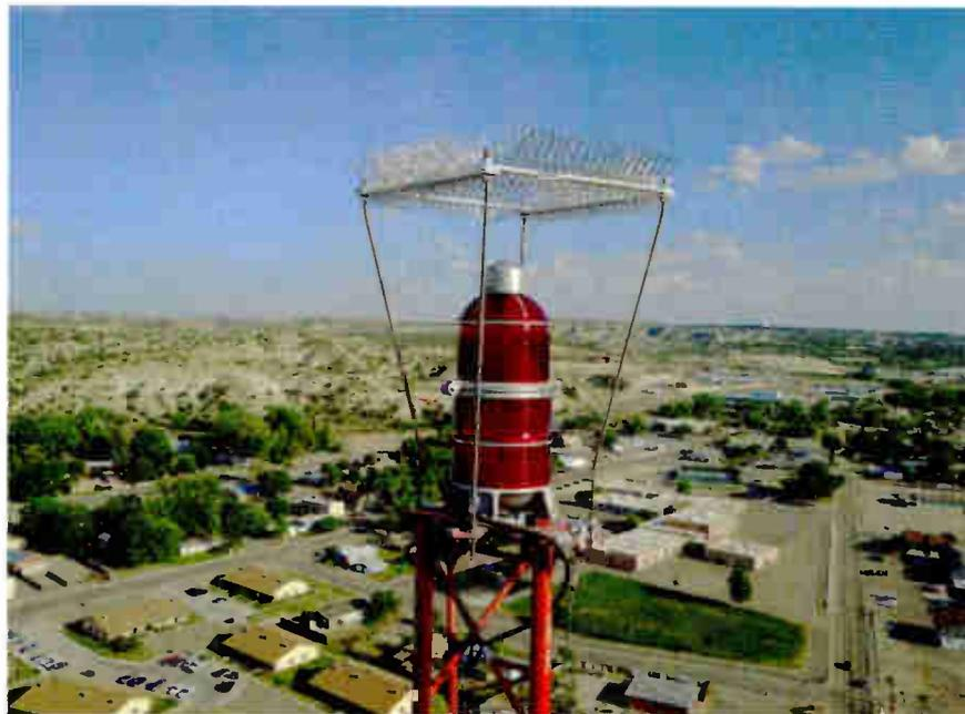
Fig. 6: A Nott static dissipater atop a tower.
