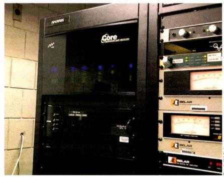
The Core64 connects WRSU's Air, Production and News studios through a single length of Cat-6 cabling. The Core64 allows operators and engineers to fine tune program source selection and intercom/talkback choices on the fly.
