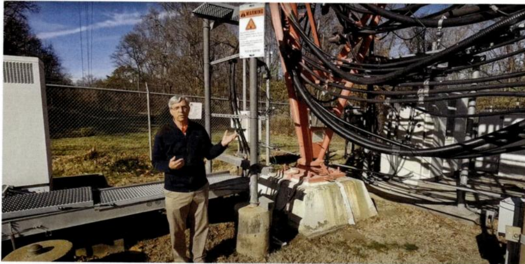
Above Joe standing at the tower base.
