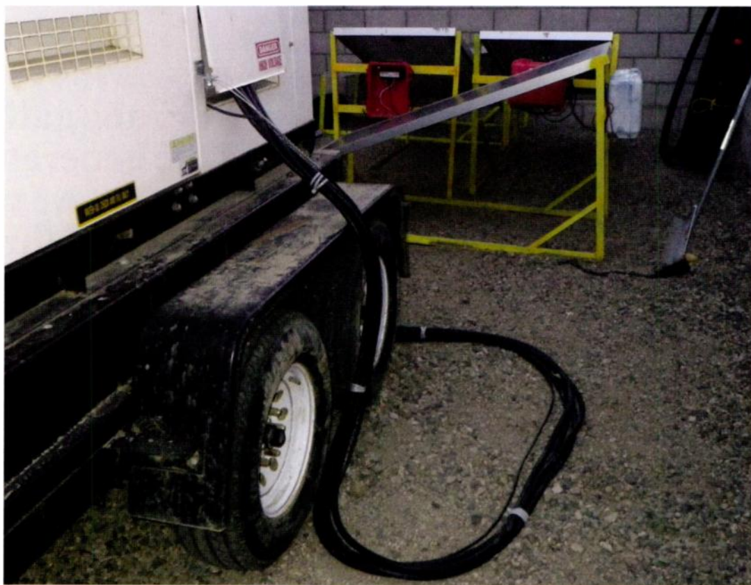
Above Power and control cables are used to connect the trailer-mounted generator.
