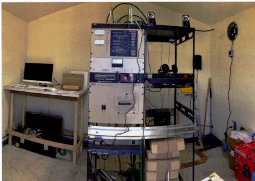
Left A fisheye view in the transmitter building during construction. Equipment includes Omnia processing, Delta ammeter, Broadcast Tools remote control, Furman line conditioner, Inovonics mod monitor and Comrex codec.
