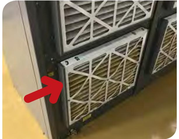
High-water mark on the filters and mud-slicked floor at KSBJ transmitter site.
