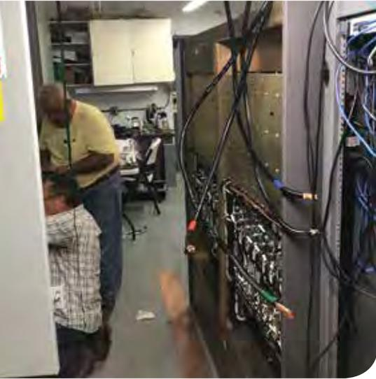
Contractors from Broadcast Site Management installing electrical wiring for the new Nautel GV40. Nautel factory personnel worked to provide a new transmitter within two weeks of the Harvey flood damage.
