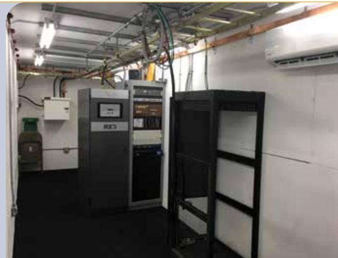
Inside the Lake Charles, LA, site. Two transmitters are yet to be moved in, one where the coax and wiring await. The other transmitter will be placed just out of frame. This installation occupies 28' of the 40' container.
