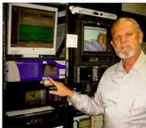
Don McKay and Ensemble Designs Avenue equipment installed at Oregon Public Broadcasting.
