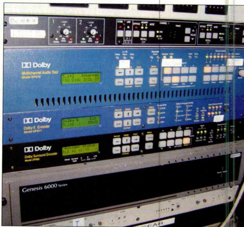
The audio program/metadata pair goes to the Dolby Digital transmission encoder, which applies the data to the appropriate stream.
