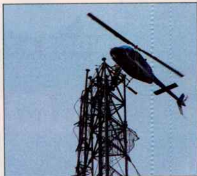
A helicopter carries a crew to reattach a portion of WPMI's tower knocked down by Hurricane Ivan.
