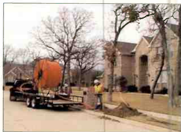
Verizon technicians lay fiber to the premises.
