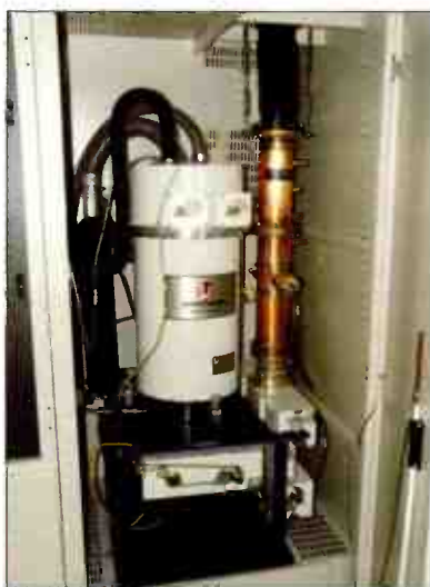
The L-3 CEA tube—an MSDC IOT—is shown here in the Thales DCX Paragon transmitter at WNEO-TV.
