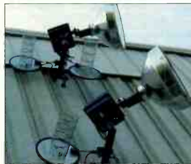
Helicals were installed both inside and outside the QVC headquarters to receive signals.
