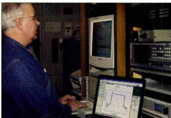
Everett Helm optimizes one of OPB's transmitters using the Z Technology DM1010.
