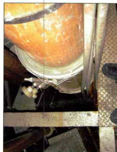
Coaxial lines and one rectangular waveguide in the mast on top of the World Trade Center, taken by the author Oct. 7, 1999.
