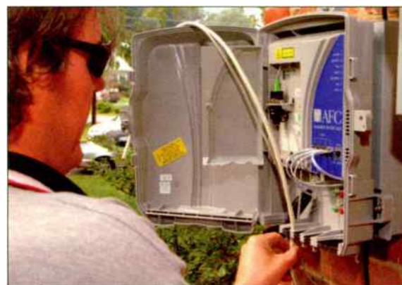
A Verizon fiber technician connects the various components of the optical network terminal on the side of a home.
