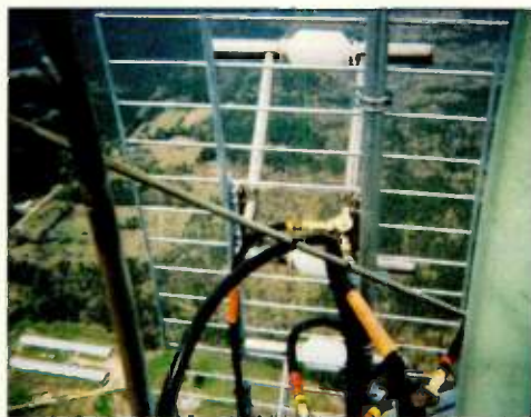
A bird's eye view of AETN's new Jampro ch. 12 antenna mounted at the 1,738-foot level of a leased tower in Huttig, Ark.
