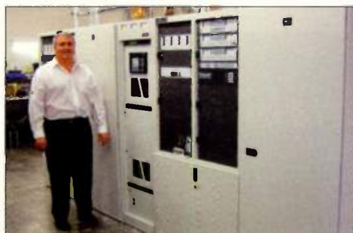
Rex Greenwell with WDSE TV/DT's new Thales Broadcast & Multimedia DCX Paragon transmitter.
