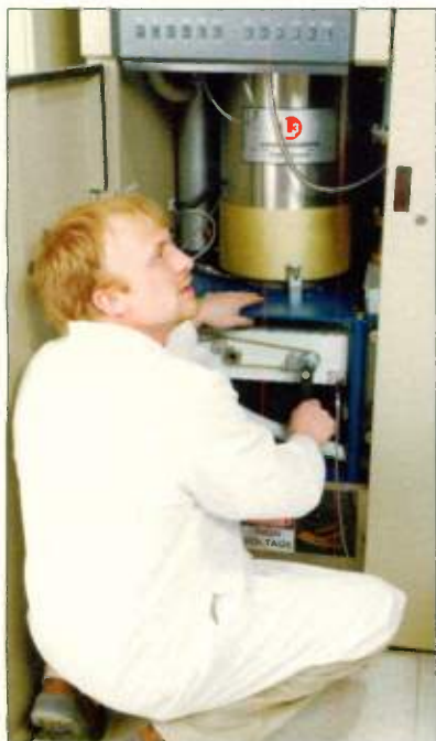
Craig Cline performs tuning operations on an IOT.
