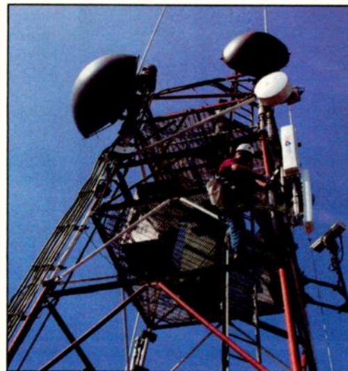
John Frercks of DSI RF Systems installs a 217 GHz system on a rooftop tower in Manhattan.
