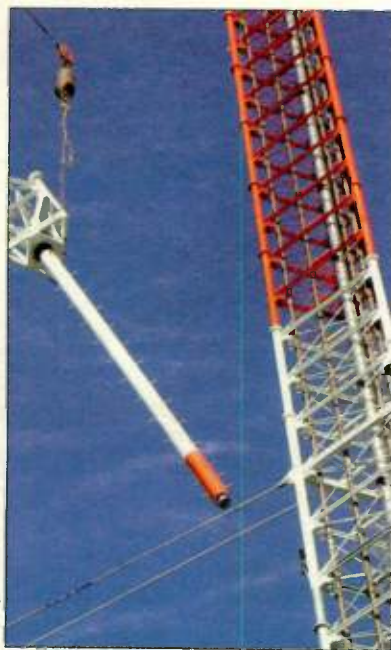
Another station is readied for digital with the installation of new antenna
