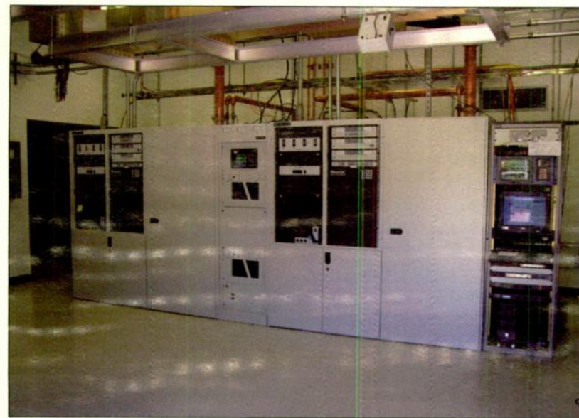
LeSea Broadcasting's WHME-DT transmission facility includes a Thomson Paragon dual-IOT transmitter.
