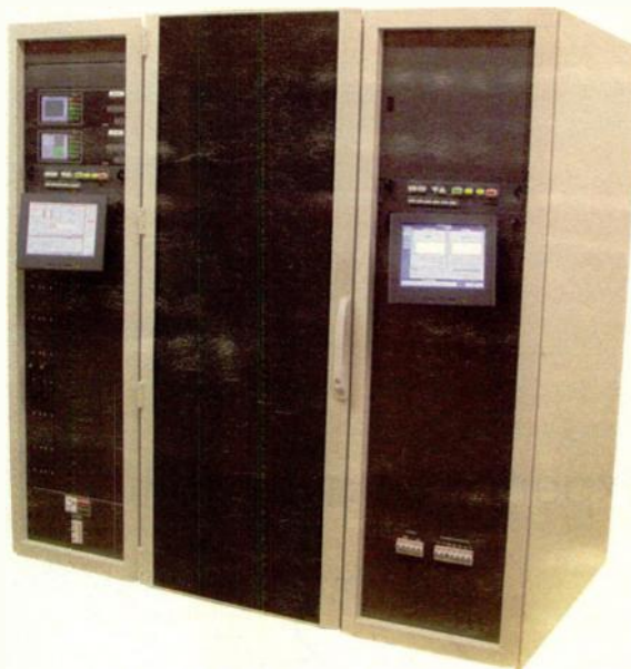
WCAX-TV uses a Harris PowerCD transmitter for its digital UHF operations.
