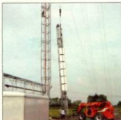
The WBSF Channel 46 PSI antenna is hoisted into place.
