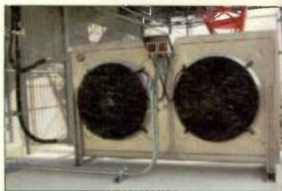
Outdoor heat exchanger used with Rohde & Schwarz liquid-cooled transmitters
