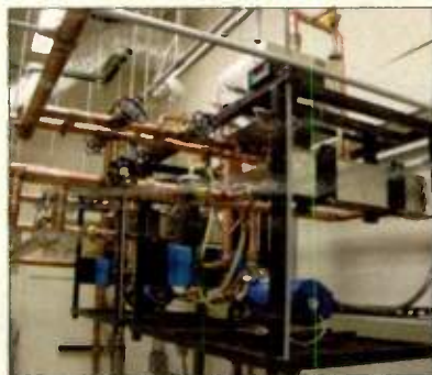
Primary pure water cooling loop used with an Axcera Visionary MSDC IOT transmitter
