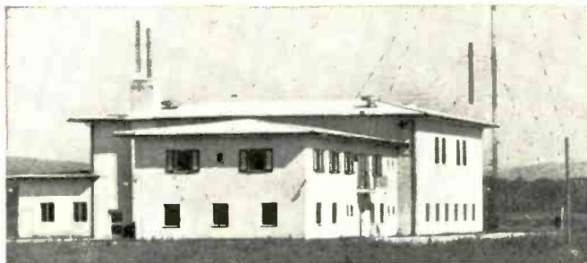
29 TRANSMITTERS like this one near Mannheim, Germany help Radio Free Europe break through the Iron Curtain. By beaming all transmitters on one target for certain periods of the day, RFE makes Soviet jamming ineffective.
