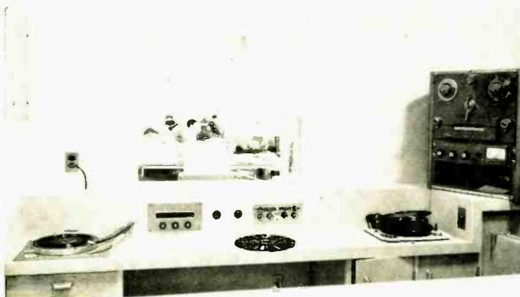
Both changer and transcription turntable play through the amplifier system in this control room. The tape recorder at the right makes it possible to record student activities when desirable.
