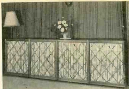
New MAESTRO, an all-horn-loaded, compression - operated uni - bass system, the world's first for home installation - gives crisp, clean and clear bass unobtainable by any cone-type woofer.
