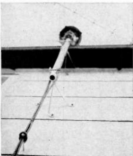
Fig. 23. Wall brackets and heavy-duty mast supporting a rotator and 10-element Yagi-Uda array. Shielded twin lead and rotator cable taped to mast and then together can be seen passing through a standoff at the bottom of the picture.
