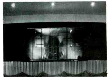
Fig. 3—Loudspeaker system appears as part of the proscenium when lights are off.
