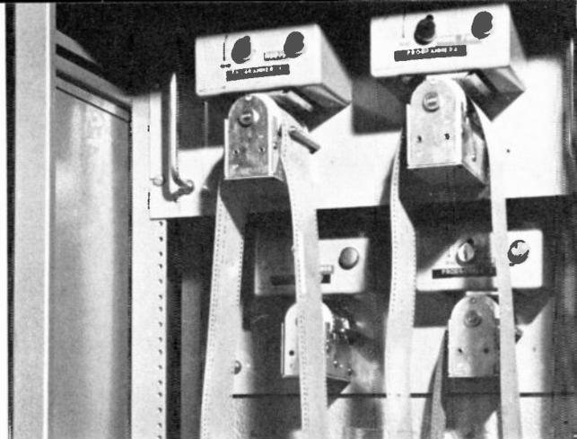
Figure 2. The control programmers for the slide projectors.
