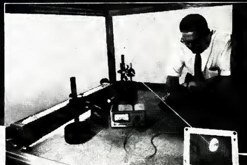
**E-V** Inside the E-V microphone laboratories is a small, dark, quiet room. And in the room is a sophisticated holographic camera. Using newly developed techniques, E-V engineers can for the first time study microphone diaphragms under actual operating conditions. Movement as small as .000005" can be seen and precisely evaluated. And this unique facility has led to new insights into microphone behavior and specifically, a brilliant new microphone design. The Model 670.
