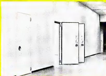
magnets, one on the door leaf and the other on the frame. The magnetic action eliminates the need for noisy latch mechanisms. Furthermore, the door can be easily opened in a panic
