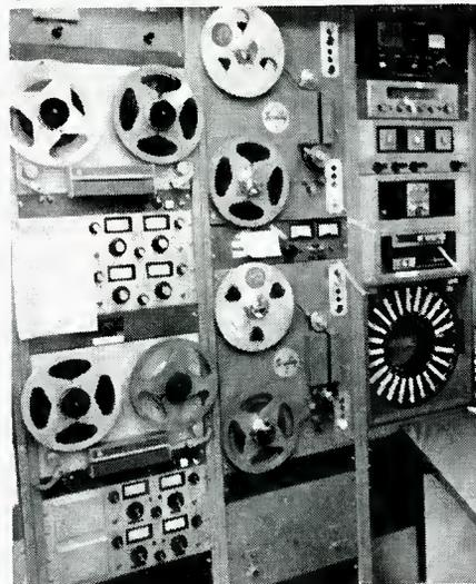
**Figure 3. The racks in control room A. Metrotech logging recorders are on the left, f.m. automation Scully recorders are in the center, and a cartridge Carousol for the automatic insert of commercials and station i.d. are on the right.**
