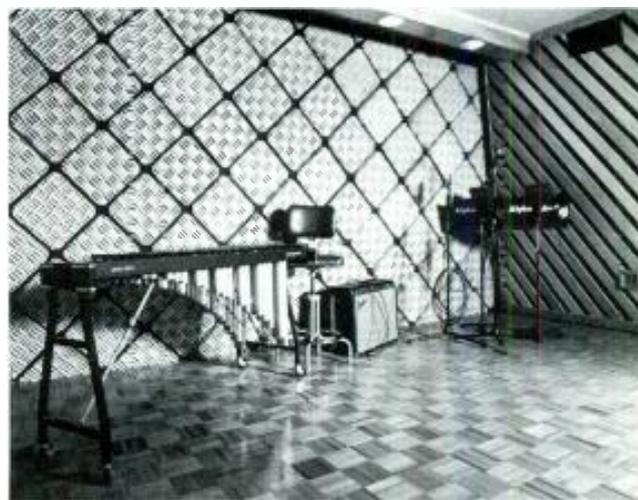
Figure 3. Audiotiles on the rear wall of Alpha's Studio IV.
