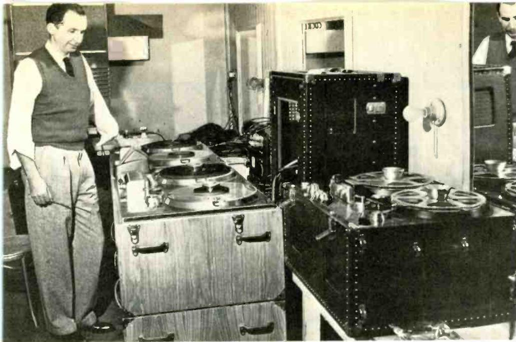
Mullin in 1950 with two "portable" Model 200 Ampex tape recorders (note the handles) and the first Model 300 to leave the factory. With these three machines, Mullin had available a full range of advanced editing techniques.
