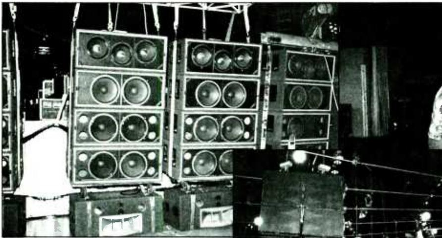
Figure 2: Nova speaker system prior to being flown at the LA Forum.
