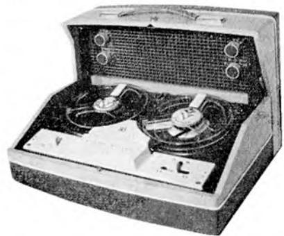
new mains recorder model 201. This is a two-speed quarter track machine using a Papst motor, with a frequency range of 40 c/s to 14 Kc/s and a price of 45 guineas.
