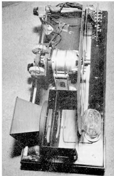
**Fig. 5 (left):** Television cabinet. Relationship viewing lens, Nipkow disc and lamp can be seen in the foreground.
