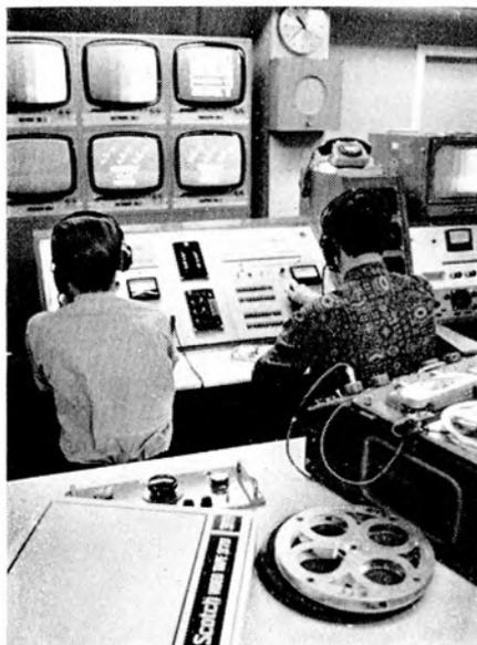
**E**DUCATIONAL TELEVISION FROM GLASGOW IN the foreground a reel of *Scotch 379* video tape and a *Series 5 Ferrograph*—not compatible. In the background, a transmission control system newly installed by *Pye* at the Television Centre in Glasgow's Bath Street. The system was built to the Educational Television Service's specification and is in use from 8.30 a.m. to 7 p.m. on weekdays. Evening educational programmes for adults will commence in the autumn.
