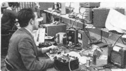
Fig. 5 Testing Printed Circuits
