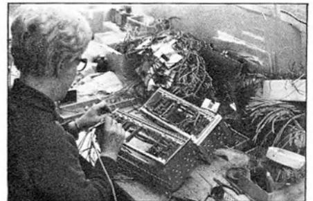
Fig. 4. Wiring circuit boards.
