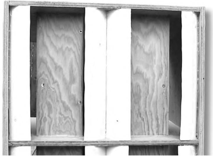
**PHOTO 19: PVC throat reflector installation.**
