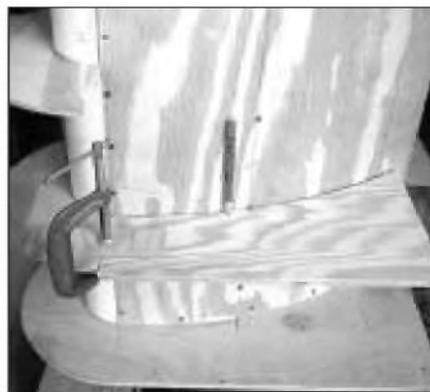
PHOTO 16: Tracing final cut line onto a side brace.
