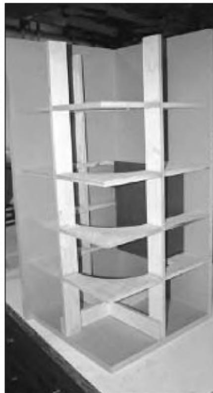
PHOTO 2: An upside down and inside view of the Extreme subwoofer enclosure showing the four shelf braces, four vertical rails, and the amplifier sub-enclosure.
