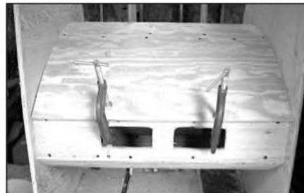
PHOTO 16: Attaching sheathing, step two.
