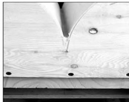
PHOTO 22: Filling the back sheath seam.
